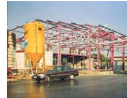
Start of construction of factory 1 (11,302 ft 2 ) in 1997
