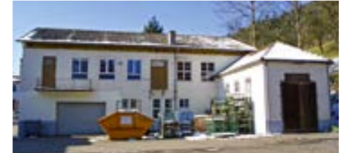
Beginnings of the suspensions factory in Klingen, 1996
